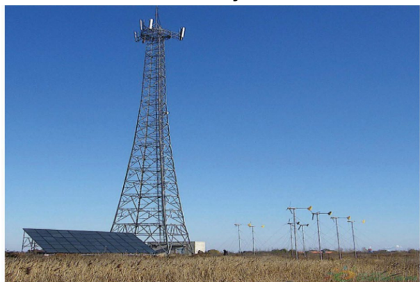
Communications base stations
