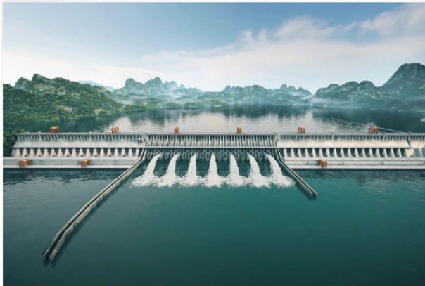
Power generation plants
